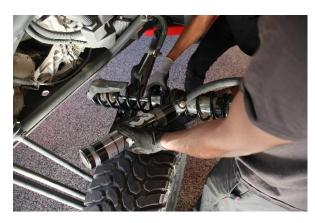
Step 5. Carefully guide the resi/resi hose through to hole in the bed, and remove coilover.
