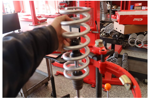
Install the Eibach tender spring.
